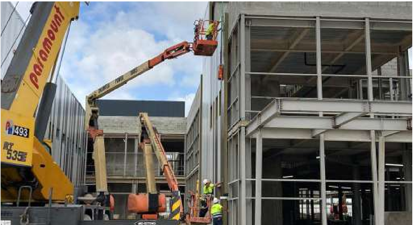
Construction of the Sangre Grande Hospital
