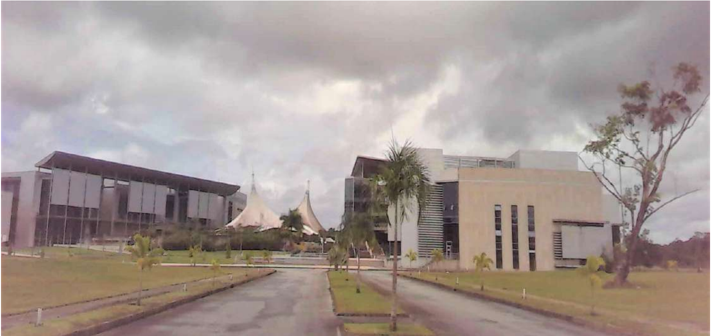
View of the UTT Main Campus East and West Blocks
