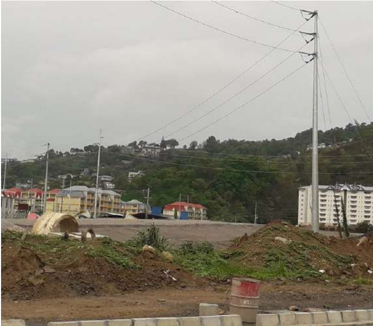
Construction of vehicular Overpass in Diego Martin
