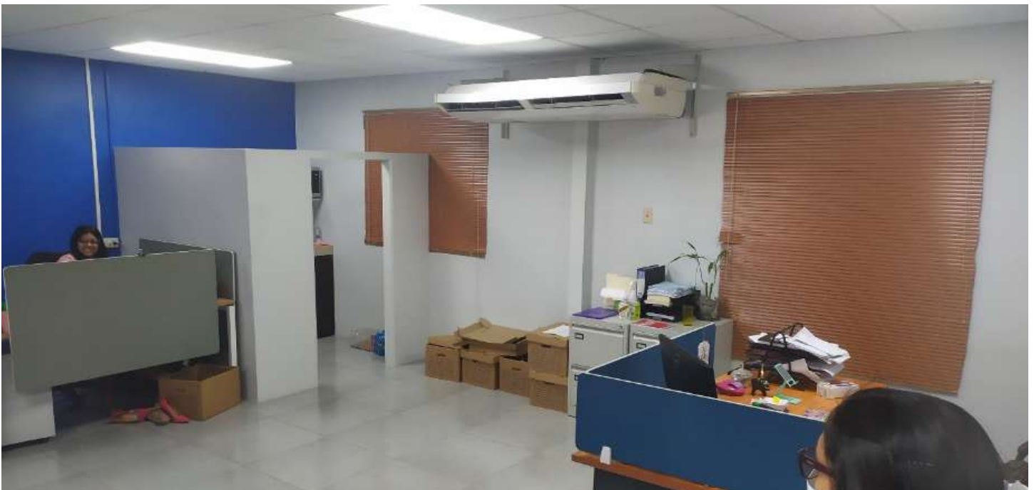
Refurbishment of the floor and ceiling - Procurement Division of PTSC
