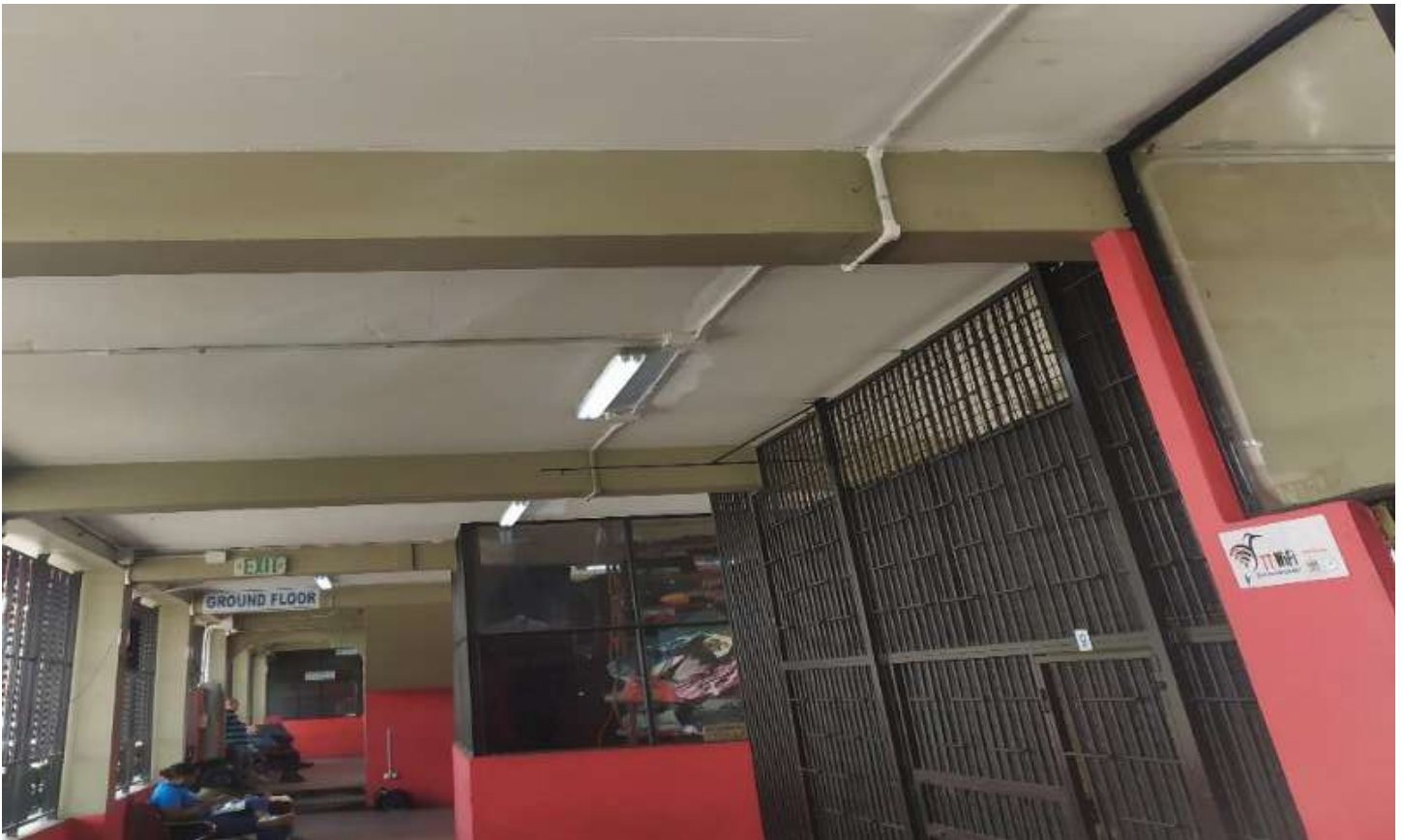
Electrical and lighting upgrade at the PTSC Curepe Transit Mall
