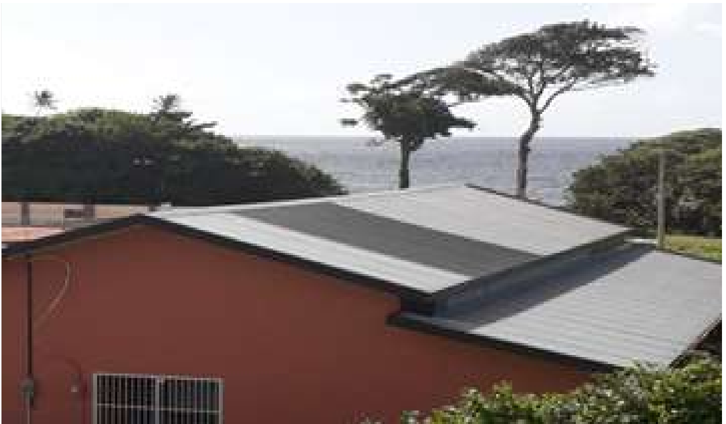
Goodwood Community Centre showing upgraded roofing
